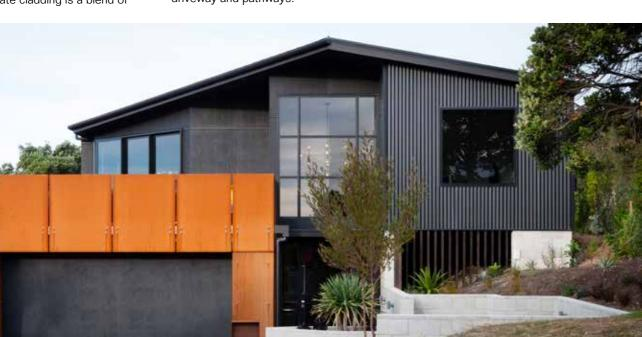
vertical Colorsteel® in Flax Pod, one of New Zealand Steel's seven new Architectural Series contemporary colours, and Shadowclad plywood panels in the deeply black Nero of Resene. The COLORSTEEL® Endura roof and all flashings, spouting and downpipes are also in Flax Pod.
