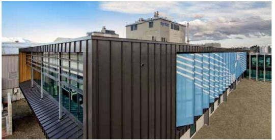
creating the seamless tray cladding. The details involved in achieving the look are very intricate, behind every tray there is a series of flashings and hooks which the tray is then folded onto, locking it into place without any visible screws or rivets. Every rib, corner and angle is carefully considered so that all of the trays line up perfectly and are spaced evenly from one corner to the next.
