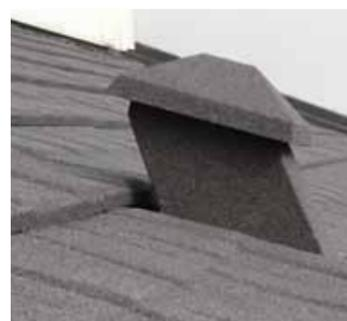
Now Metrotile in New Zealand announces it is to supply J.A. Plast vent tiles to go with its metal tile roofs in New Zealand. These will be of two types – one to ventilate the roof space and allow air introduced at the eave to escape carrying with it moisture which can otherwise cause "leaking" issues. The
