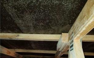
Prolonged wetness of underlay and structure can result in mould growth. This is often initiated in the post-enclosure building stages of a contract.
