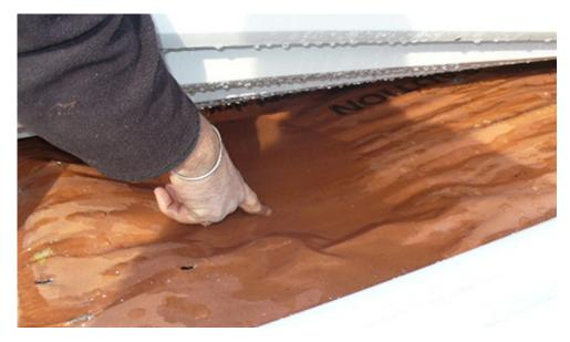
Once all absorbent surfaces are saturated, condensation can pool on the upper surface of the roofing underlay. It is the result of a gross imbalance between water vapour entering the ceiling cavity and water vapour escaping.
