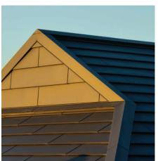
Calibre was designed with performance in mind, making it ideal for a location like Mt Maunganui, which endures heavy wind-driven rain and exposure to harsh winds. Calibre utilises a Concealed Fastening (CF) design, which conceals fasteners by hiding them underneath an interlocking nose-to-head lapping method. This creates a strong matrix of panels, protected against wind and water ingress, delivering high functionality in an environment that demands it.
