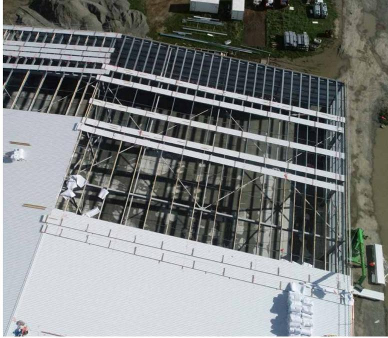
Sheets in lengths of 38.810m posed the first problem – production of this length would extend several meters outside the parameters of the factory, creating the need to have the product produced, loaded and exiting the factory in a single workday.
