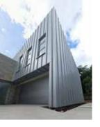
We started the roof pitch at the low end, about 3 degrees, and at every rafter we increased the pitch slightly until we reached 25 degrees at the high end creating a subtle twist.
