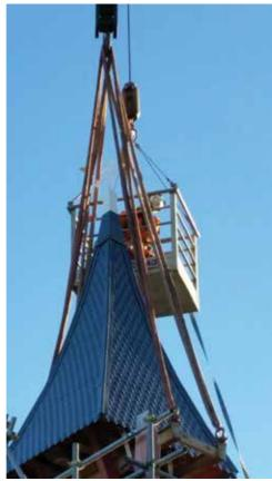
decay present in some of the timber members both within the belfry and the church below and the decision was made to remove the belfry for repair and restoration. The belfry was craned off the building and both it and the church were repaired, both no small feats.
