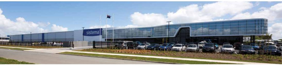
The structural grid design of the building was based on the size of the machinery it had to accommodate for the production line and gantry cranes. A mixture of traditionally reinforced, fibre reinforced, combislab and post-tensioned concrete floors with epoxy coatings were used to meet the varying demands of the facility.
