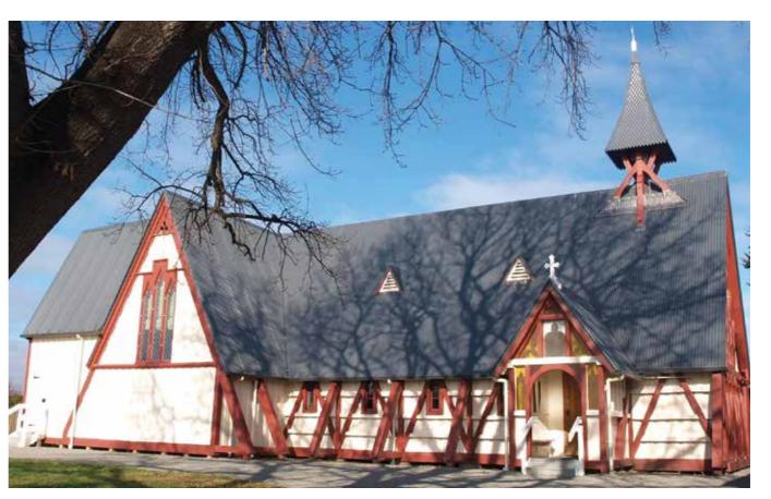
"The lead flashings on the belfry are a work of art and well worth preserving despite the possible drawbacks", says Suzanne," and considerable care was taken to isolate the two metals as far as possible".
