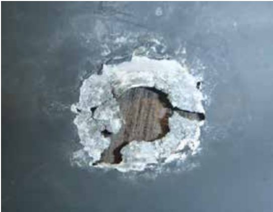
Painted aluminium corrosion due to contact with stainless steel fasteners. Pinhole corrosion was also evident within 150mm of many fasteners.
