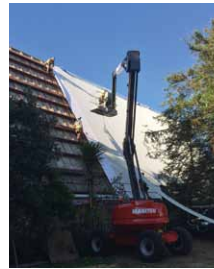
20m aerial work platform was purchased specifically to work on the 80% roof pitch
