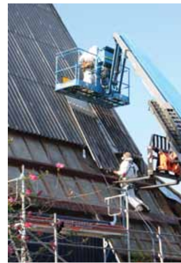
Specialized safety clothing and techniques were required to ensure asbestos fibres were not released during the roof removal process
