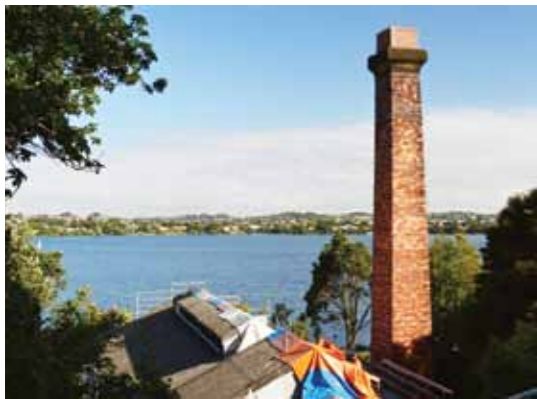
Part of the project required the removal of the asbestos roof. The removal, disposal and spray treatment was carefully monitored.
