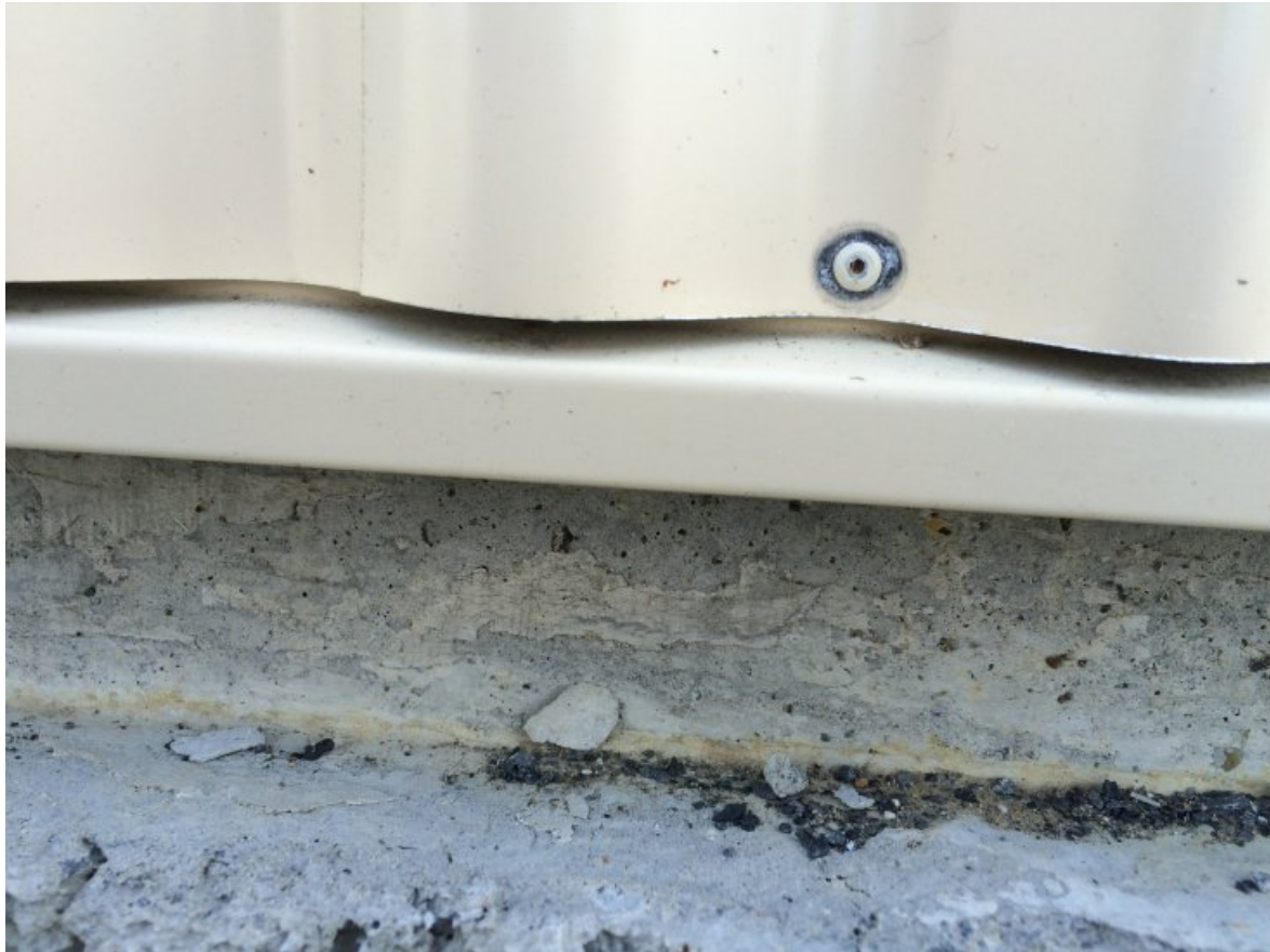
Stainless rivets will cause corrosion to Z AZ and ZA-coated products.
