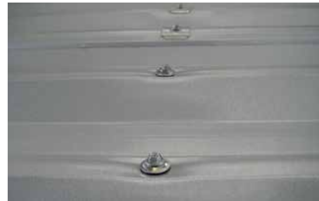
Typical serviceability failure. Distortion around fastener lead.
