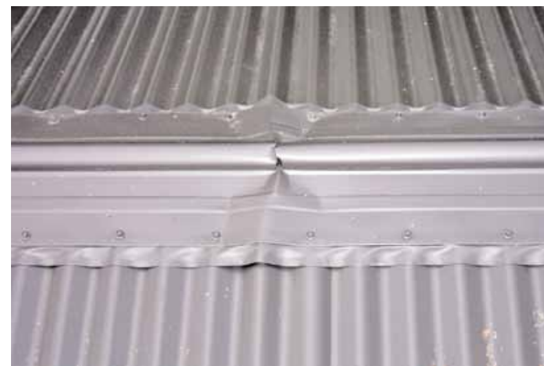
Figure 2 Buckled change of pitch flashing
